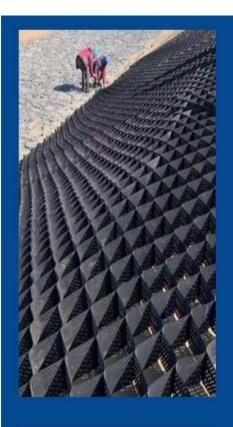
Geogrid is a geosynthetic material used to reinforce soils, retaining walls, sub-bases, and subsoils.
